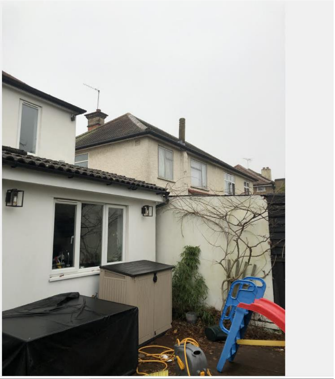
View of No. 33 from host property garden
